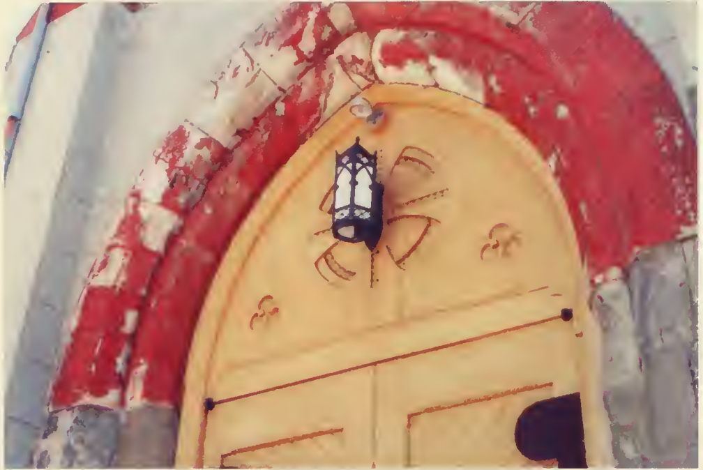
North Elevation of Church Building (J)
